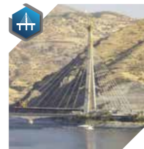
Kömürhan Bridge, Turkey
