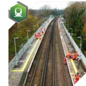
West Dulwich Station, UK
